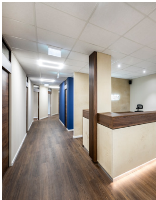
The practice premises are heated and cooled via ceiling convectors – space-saving, efficient, and without conventional radiators.
